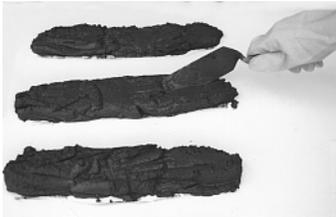
For each hearth slab, place three rows of mortar (2" apart), approximately 3" (7.62cm) wide and 3/4" (1.91cm) thick.
