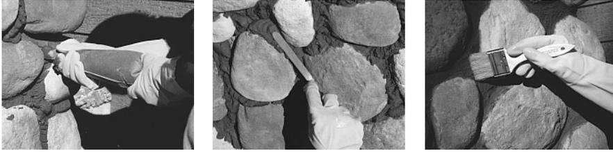
2. When mortar becomes partially firm, compact the joints and level them off with a jointer. For the final finishing, brush joints with a dry paint brush.
